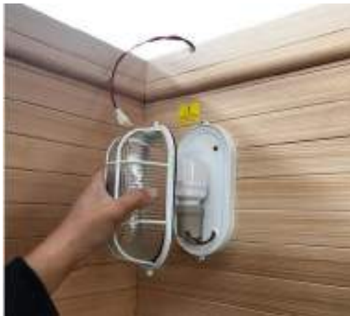
13 Install sauna lights waterproof cover, just use screws, see above photo glass screws M3x20mm
