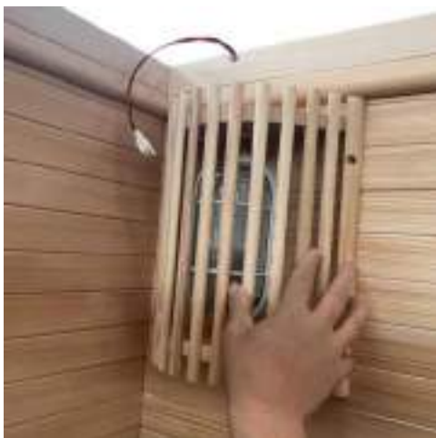
14, Assemble wood cover for sauna lights , USE Screw 3.5x25
