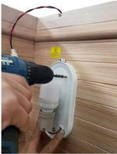
12. Use screws to fix the sauna light pedestal, see above glass screws M3x20mm
